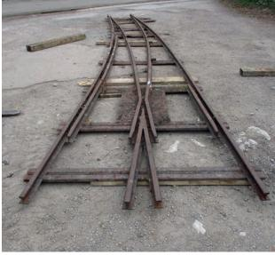
Item 31 R/H turnout, 20lb/yd rail, 16'6"ft long, approx 1 in 4 angle. Welded to rail section sleepers. Rough condition.
